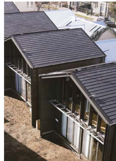
BELOW The new roofs under construction
